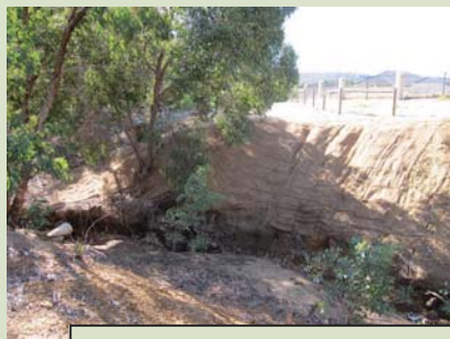
Jute matting applied to prevent erosion
